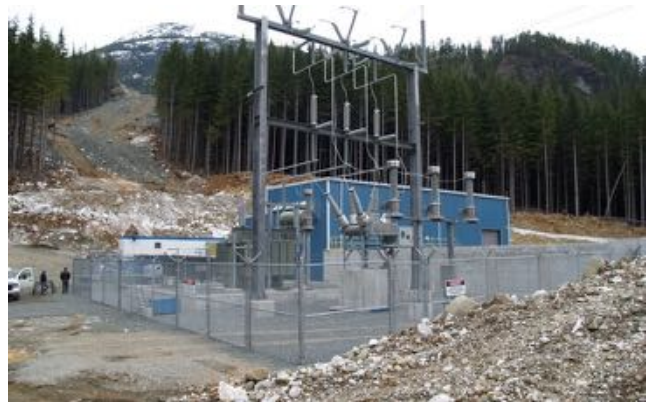
Zeballos Hydroelectric Project
